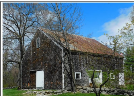
The Barn – Gifted to the Town 2018 – Dismantled Spring 2018
